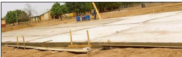
The completed foundation!
