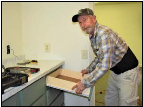
Darrell McGinty setting cabinets and countertops, and adjusting drawers
