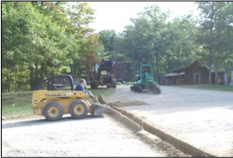
Dale Jones and Crew installing the fiber
